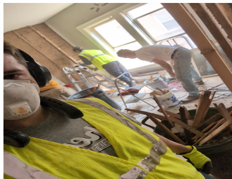
Did some volunteer demolition for the ICCM Life Center
